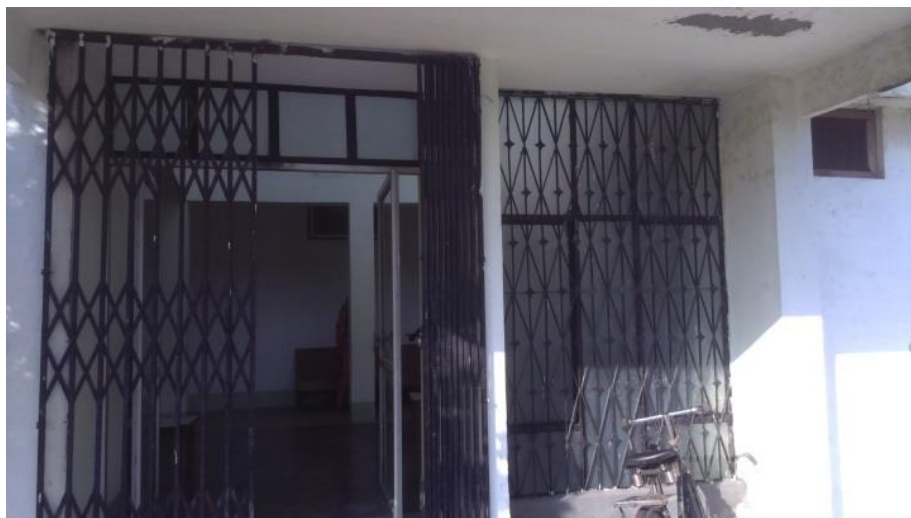
Figure 3: Entrance to the property
