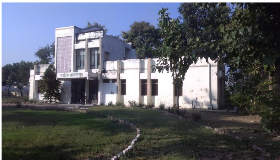
Figure 2: Main building in the premises
